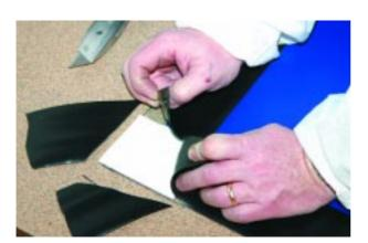
**Step 5.3**Mitre the corners and secure onto the Edging Tape
