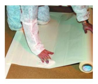
Step 2.1 Sweep the area again, then lay out the metre wide tape to cover all of the area inside of the Edging Tape
