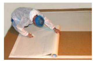
**Step 2.2** Laying the metre wide tape where one or more strips are needed.
