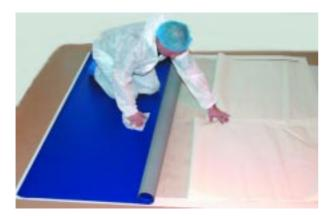
**Step 3.2**Removing backing paper from metre wide tape and laying material
