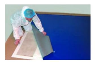
**Step 3.1**Rolling back material to remove the backing paper from the metre wide tape
