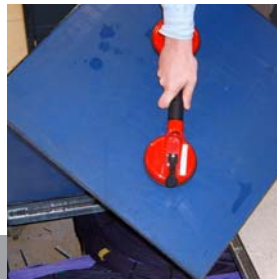
Dycem can be installed on individual access tiles or directly onto the floor substrate.
